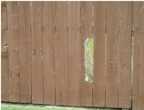
Damaged picket
