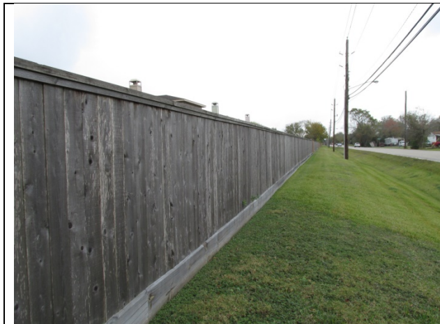
Overview of fence by Miller Ranch Road
