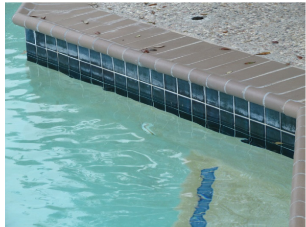
Efflorescence
