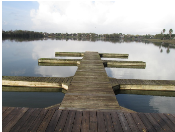
Floating docks overview
